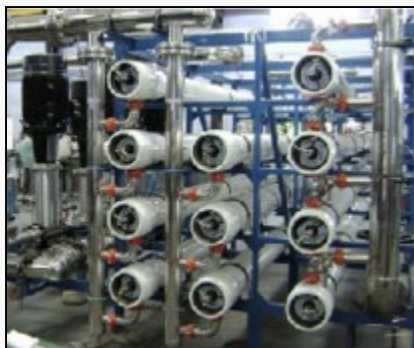
Recycle & Reuse - Membrane Based System
