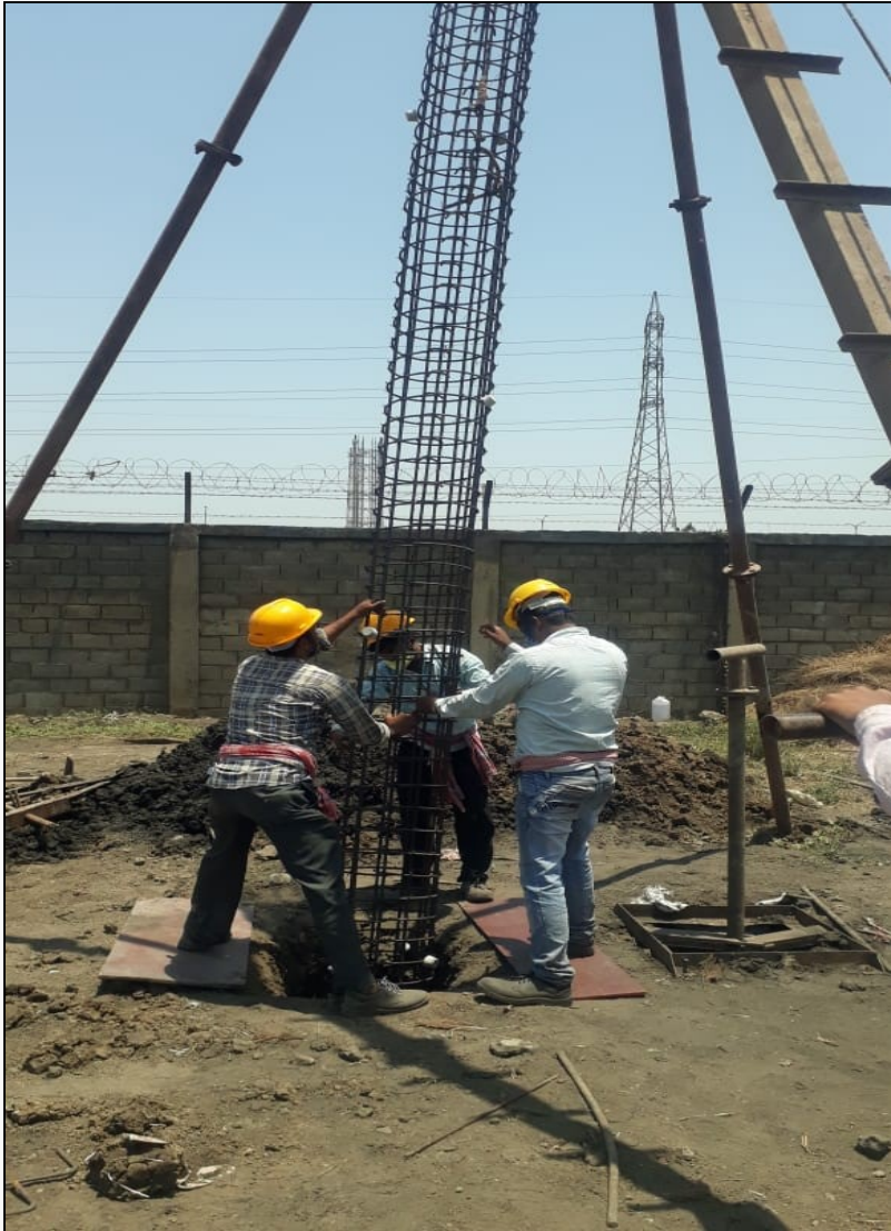
Piling Works at GFL, Dahej
